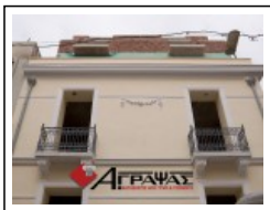
Reconstruction of neoclassical residence Reconstructions Oct '10
