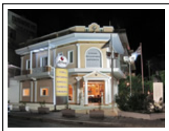
A.Grapsas LTD - Alimos Store Offices/Stores Jul '00
