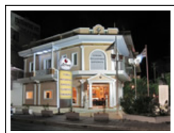
A.Grapsas LTD - Alimos Store Offices/Stores Jul '00
