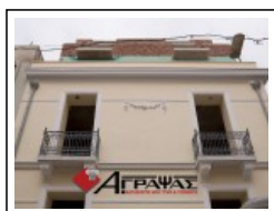
Reconstruction of neoclassical residence Reconstructions Oct '10
